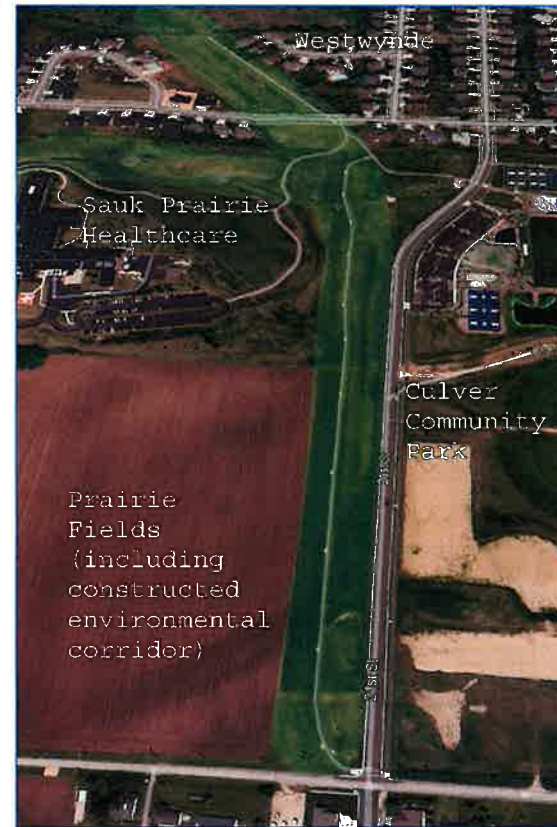
Environmental corridors on Prairie du Sac’s western edge have been established with development of adjacent lands, graded and vegetated for stormwater infiltration and movement, and outfitted with trails for passive recreation. (Image Google Earth, 2025)
